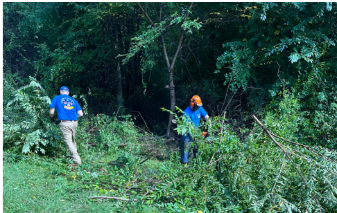
Brush Clearing at Dellinger Lodge
