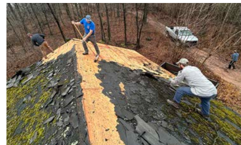
Replacing Roofs at Ford and Snavelly Pavilion
