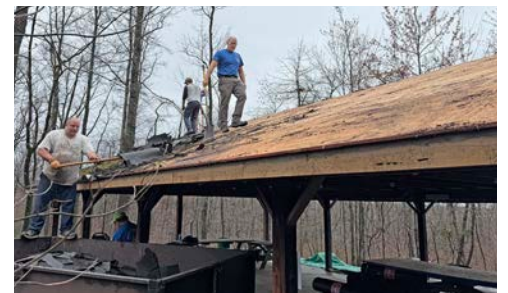
Replacing Roofs at Ford and Snavelly Pavilion
