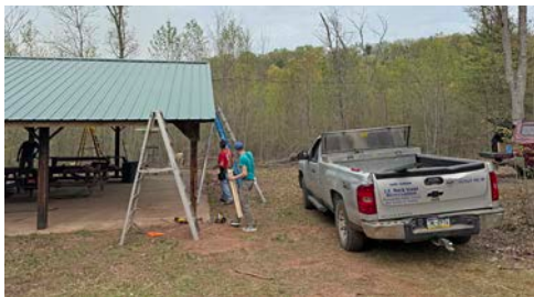
Snavely Pavilion Roof Work
