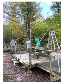
Starting Chippewa Demolition
