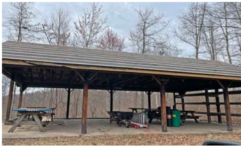
Ford Pavilion Roof Work
