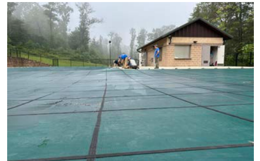
Installing Pool Cover for Winter
