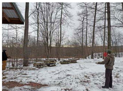
Laying out new campsite design
