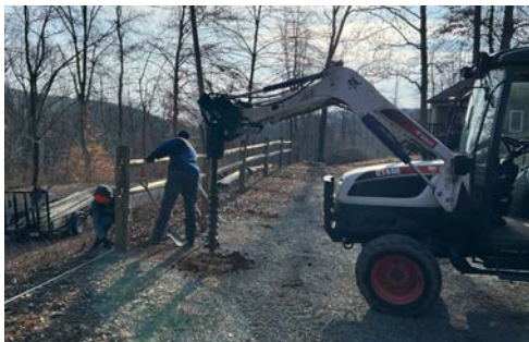
Installing Fence at Training Center
