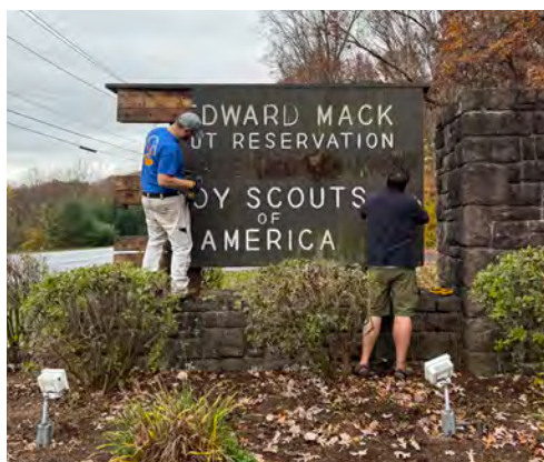
Demolition of the old Camp Mack sign
