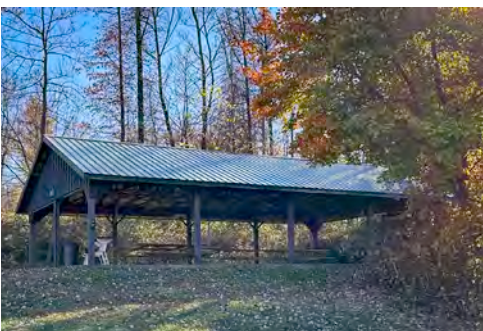
New Metal Roof on Hyman Pavillion
