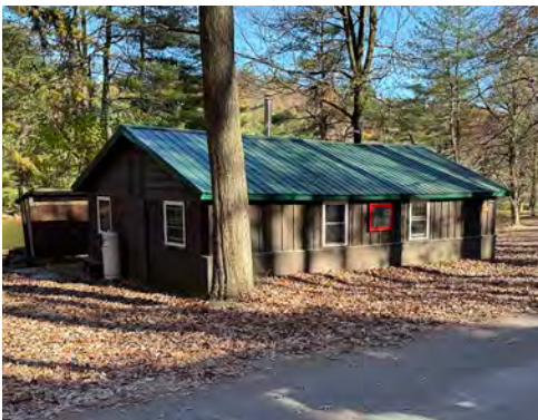
New Metal Roof on Swarr Lodge
