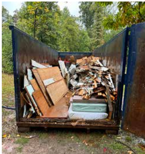
Old Health Lodge interior demolition
