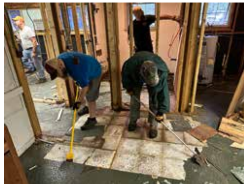
Old Health Lodge interior demolition
