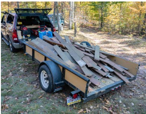
Bottom photos: A contingent of Friends begin dismantling the Cherokee campsite platforms.
